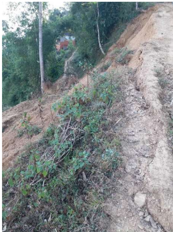
Photo:14 Landslide at Nayagaun
