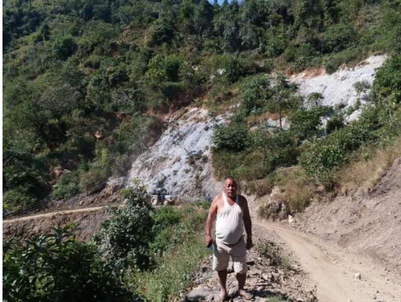
Photo:13 Landslide at Dhuwa Khola
