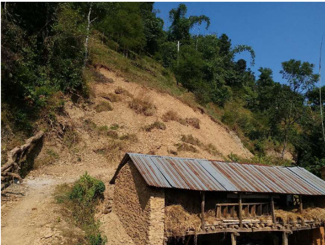
Photo:11 Landslide at Urleni Gaun
