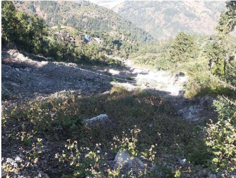
Photo:3 Landslide at Nigare village
